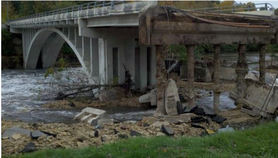
**September 2010:** Heavy rain fell towards the end of September on abnormally wet soils, resulting in significant river and flash flooding. The approach on the north side of the County Road 18 bridge going through Oronoco washed out (Figure 14), due to the Zumbro River flooding
