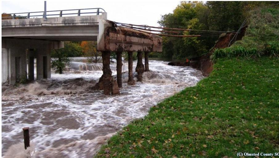
During the 2010 floods in Oronoco, the Lake Shady dam gave out and flooded the city (Figure 25), destroying the lake in the process, as it eventually turned into a sediment-filled floodplain. The dam was removed in early 2017 by Olmsted County Environmental Resources, and the river
