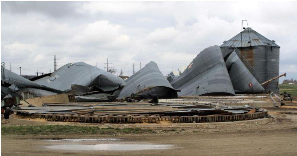
In March of 2012 severe storms produced high winds which ripped the lids off four 50,000-bushel galvanized steel bins and pushed them over (Figure 10). An empty 30,000-gallon fuel tank was also toppled, and some grain semi-trailers
