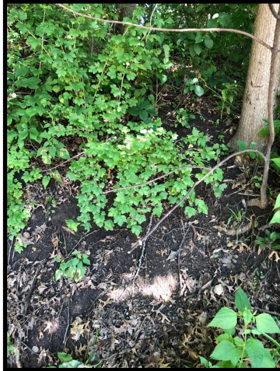
Figure 3: Photograph of Existing Slope Conditions in Western Project Area. Facing West.
