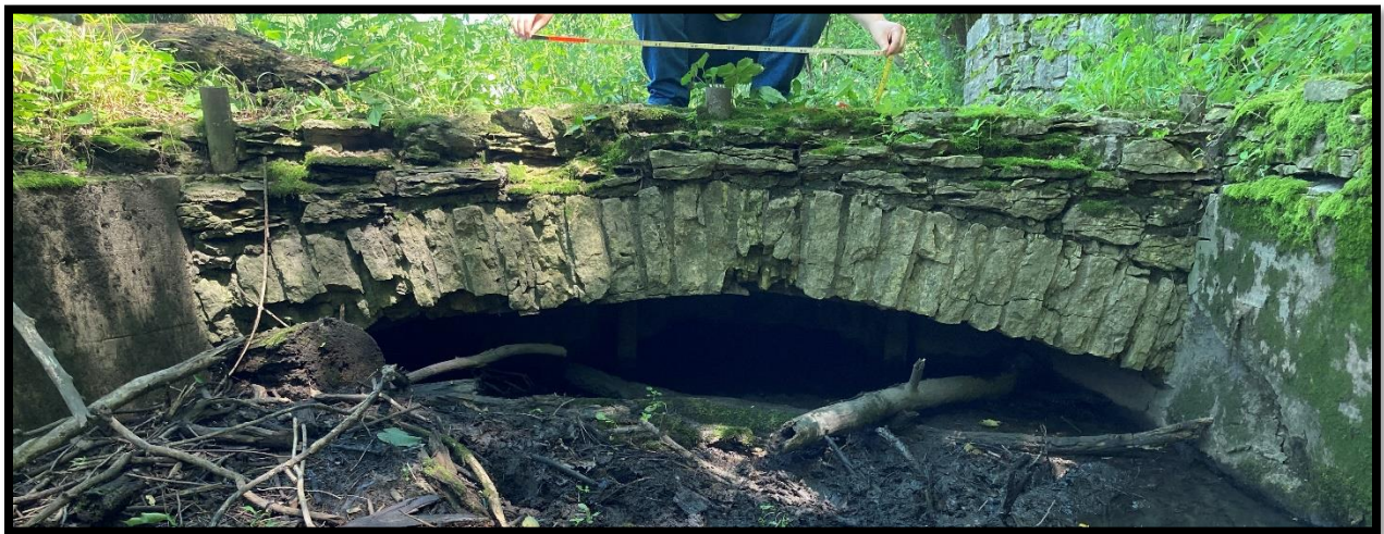
Figure 7: Eastern Entrance of Concrete and Stone Water Control Feature.
