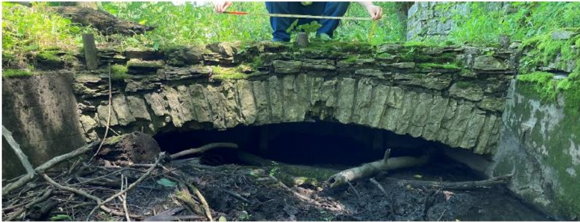
Figure 8: Eastern Entrance of Concrete and Stone Water Control Feature (with a one-meter tape for scale).
