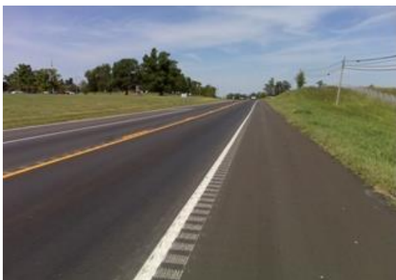
Edgeline Rumble Strips
