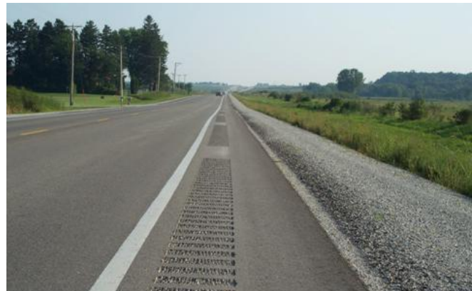
Shoulder Rumble Strips
