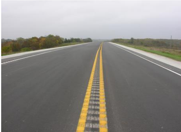
Figure 3-5. Centerline Rumble Strip
