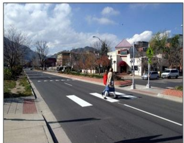
Figure 3-10. Center Island Medians (Pedestrian Refuge Island)
