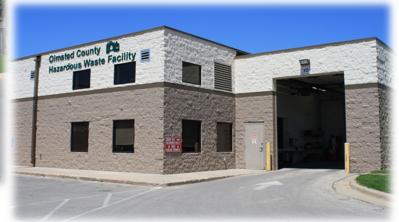
Hazardous Waste Facility
