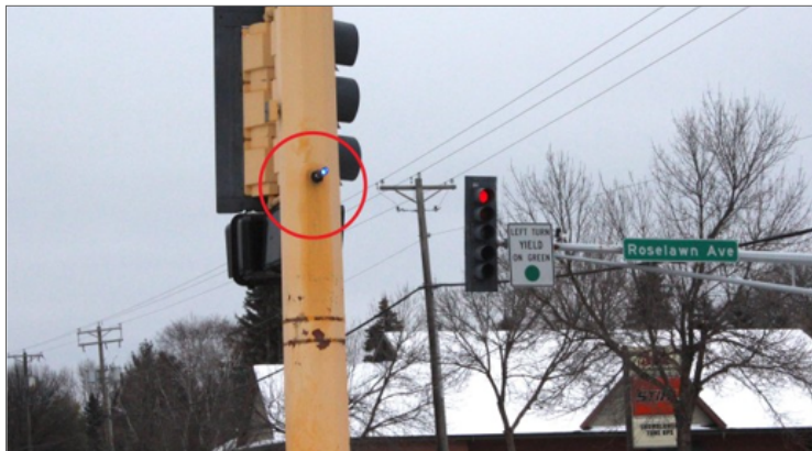
Figure 2: Blue confirmation light on signal system
