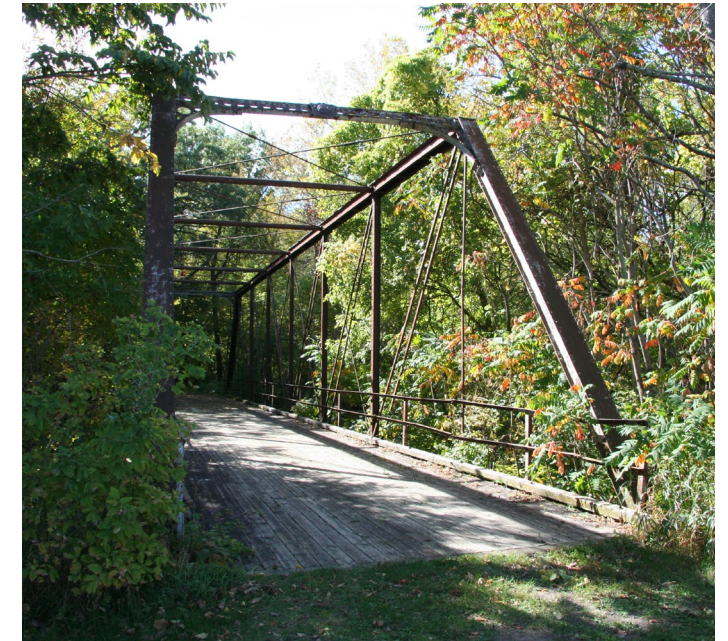
BRIDGE 4846 – 1875 VERNON BRIDGE LE SUEUR COUNTY
