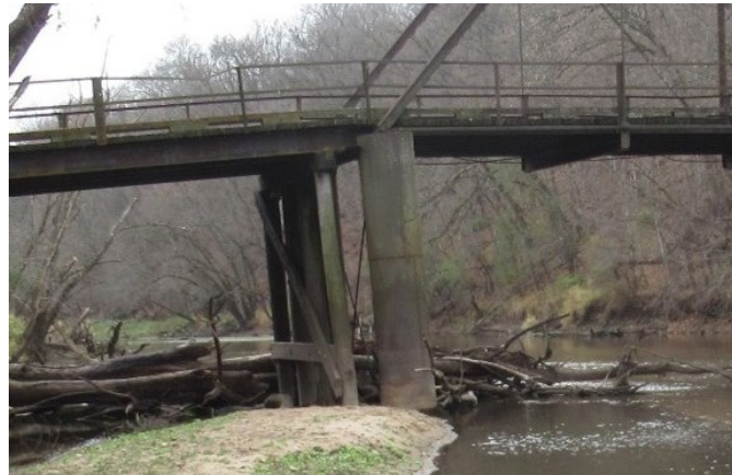
East Truss Pier
