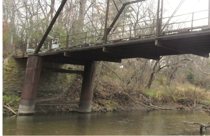
West Truss Pier
