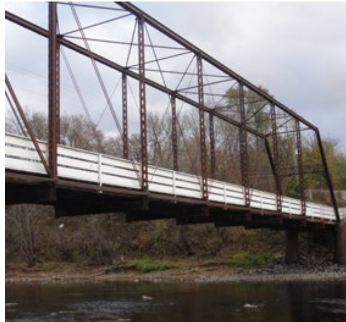
BRIDGE 92366 – 1885 HANOVER BRIDGE WRIGHT COUNTY
