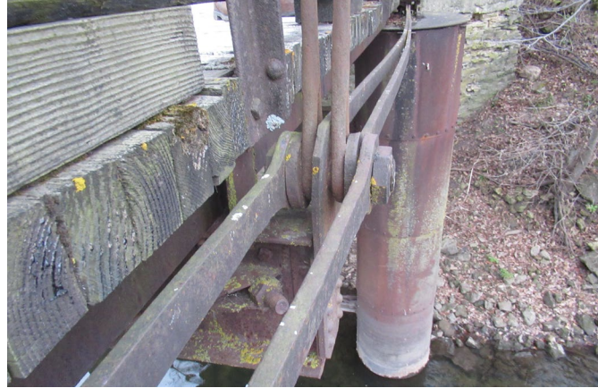
Seized Pin & Warped Chord
