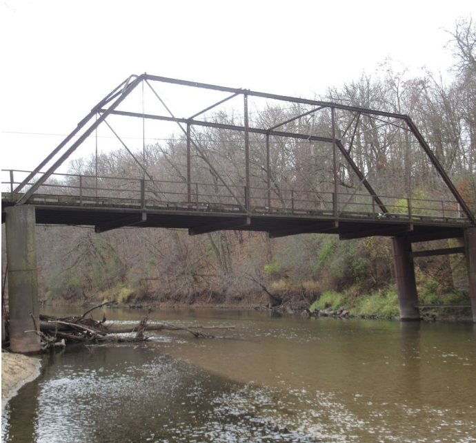
BRIDGE L6322 – 1895 FRANK'S FORD BRIDGE OLMSTED COUNTY
