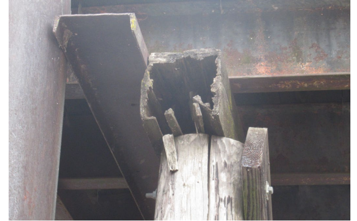
Timber Pier Cap
