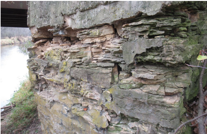
West Stone Masonry Wingwall
