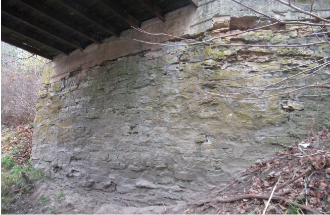
West Stone Masonry Abutment
